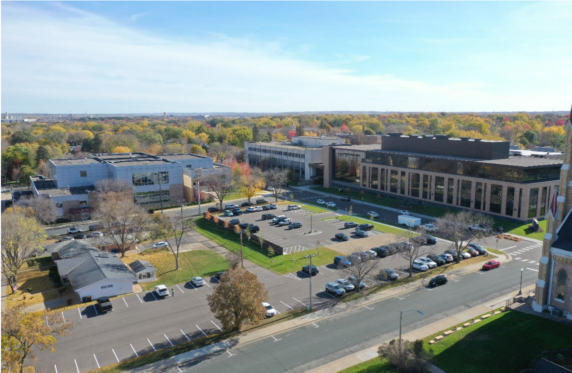
Photo: Scott County Government Center Campus, Shakopee, Minnesota
